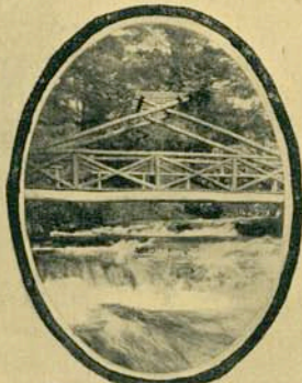
The Upper Bridge
