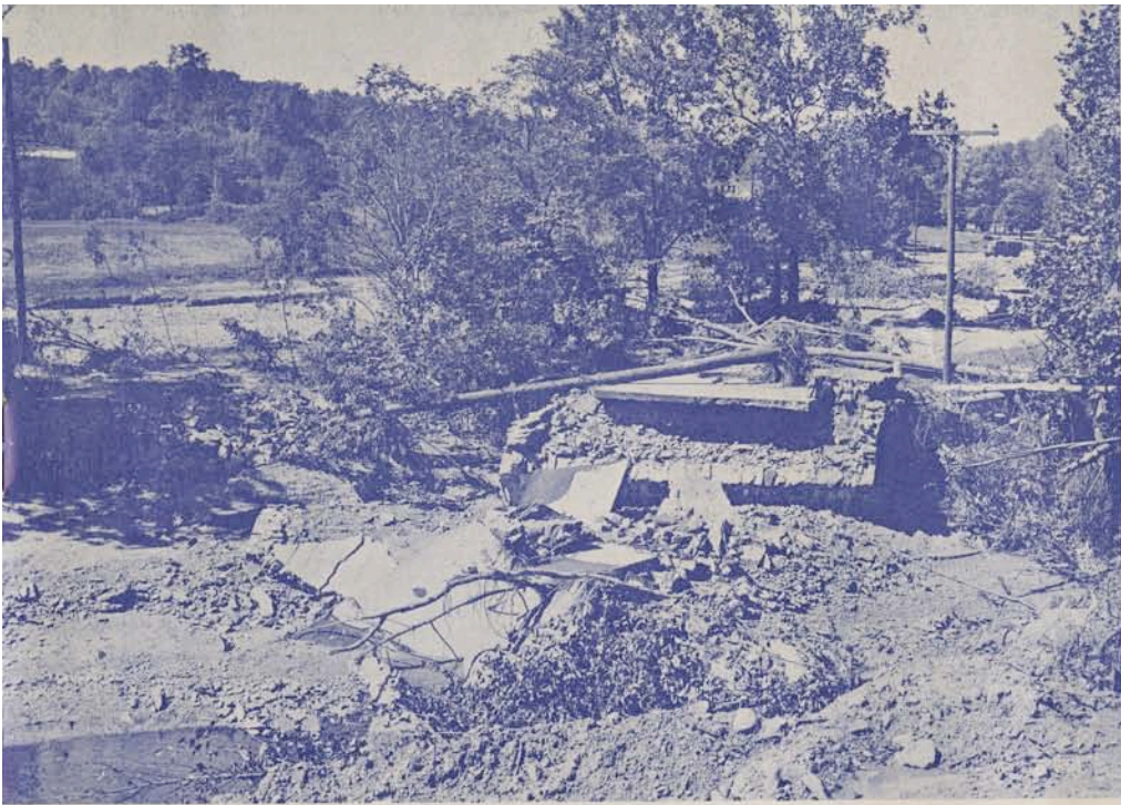
ANALOMINK CREEK, Henryville. Traffic Route 90. 64-foot span replaces old masonry arch destroyed by raging creek.
