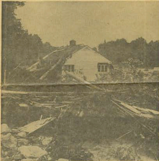
SHATTERED SUMMER HOME —Nearly every home in Canadensis received a battering from the flash floods in that area. But this home, surrounded by huge piles of debris, received one of the severest hammerings. Lifted from its foundations and carried away by swirling flood waters, the home is now high and dry—but visitors will need a bulldozer to get inside.
