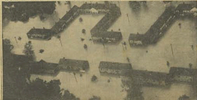
The Dauntless Lane Apartments at Hartford, Conn., live up to their name as they stay on their foundations despite 10 feet of flood waters. Several hundred tenants were evacuated, however.
