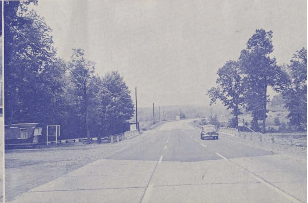
POCONO CREEK, north of Bartonville. Traffic Route 611. Replacement of 45-foot concrete bridge by 64-foot span permits major improvement of alignment and approaches.
