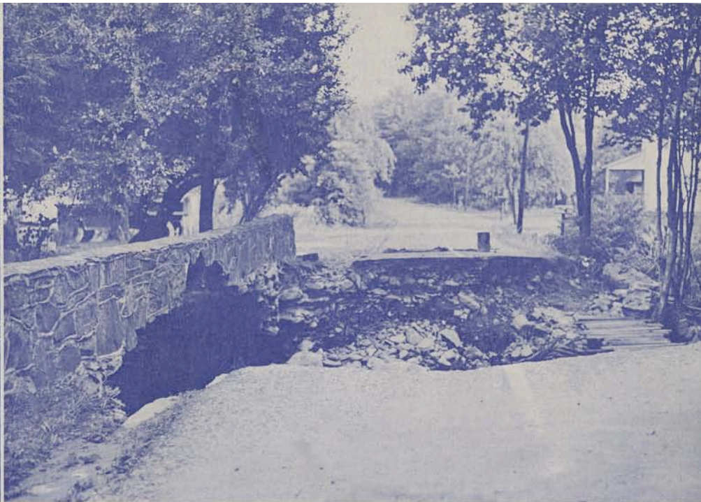
BRODHEAD CREEK, Covesville. Traffic Route 290. Masonry arch being replaced by concrete 50-foot span. This job has been completed and road is in full service.
