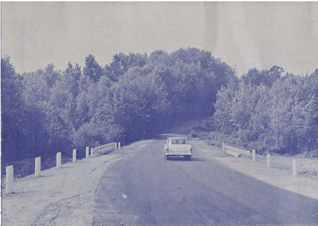
FOREST HILLS CREEK, Swiftwater. Legislative Route 45034. 24-foot concrete span replaces 15-foot masonry arch.
