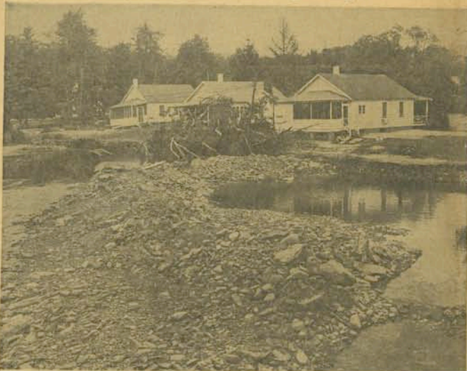
SUMMER HOMES SMASHED —Three pleasant summer homes in Canadensis were raked by turbulent flood waters of Broodhead Creek. After the waters receded the owners found their homes uprooted from foundations and encased in a pile of rocks, trees and other debris. In center of picture is retaining wall erected to enclose the creek.
