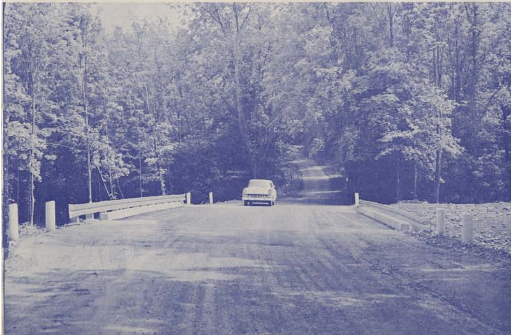
PARADISE CREEK, Henryville. Legislative Route 45025. 18-foot span replacement for masonry arch.
