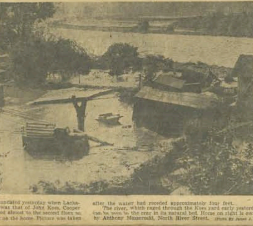
One of the homes in Duryea inundated yesterday when Lackawanna River went over its banks was that of John Koytek, Cooper Street. Water from the river reached almost to the second floor so far as can be seen by the black mark left on the house. Picture was taken after the water had receded approximately four feet.
