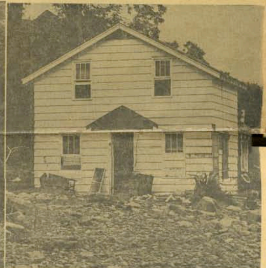
TYPICAL SCENE IN CANADENSIS —This is one of many homes in Canadensis which fell prey to angry flood waters of Broodhead Creek. This home, owned by Joseph Simons, was lifted off its foundations and carried at least 75 yards away. Rocks and trees combined to splinter the roof and ceiling.
