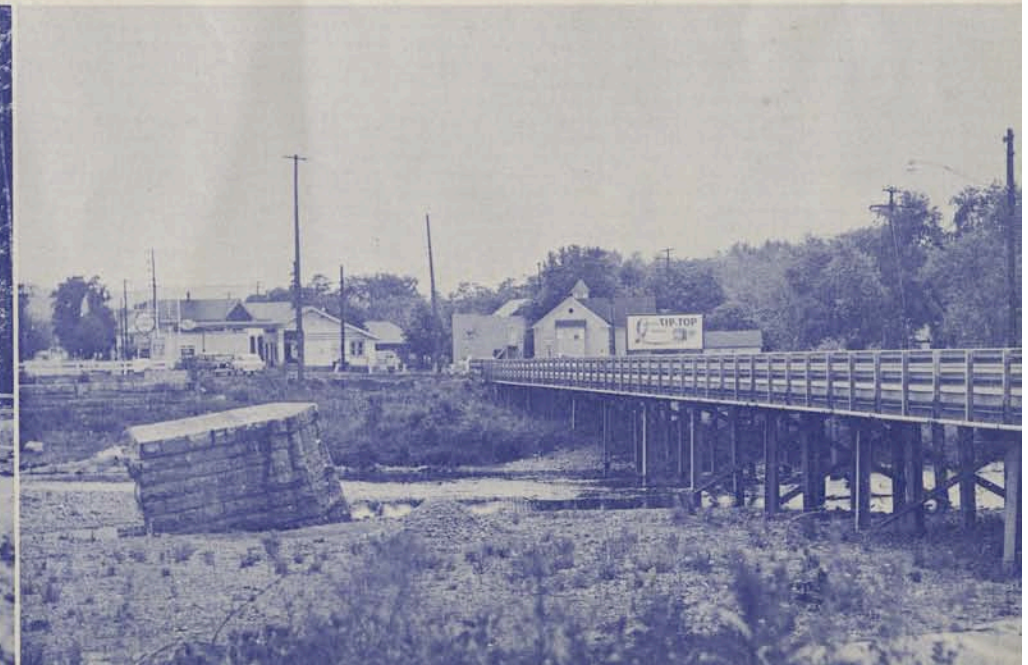
BRODHEAD CREEK, connecting Stroudsburg. Off Traffic Route 611. Old bridge completely destroyed, replaced by temporary structure shown above, while new modern bridge is being designed.
