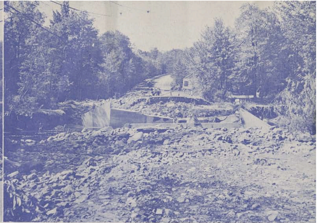
TOBYHANNA CREEK, west of Blakeslee Corners. Traffic Route 940. Nearing completion is two 68-foot span concrete bridge replacing old two 48-foot span which was destroyed.
