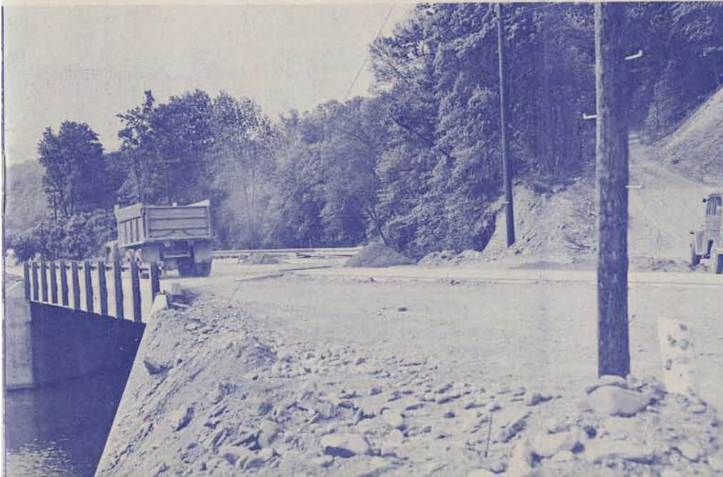
ANALOMINK CREEK, Henryville. Traffic Route 90. 64-foot span replaces old masonry arch destroyed by raging creek.
