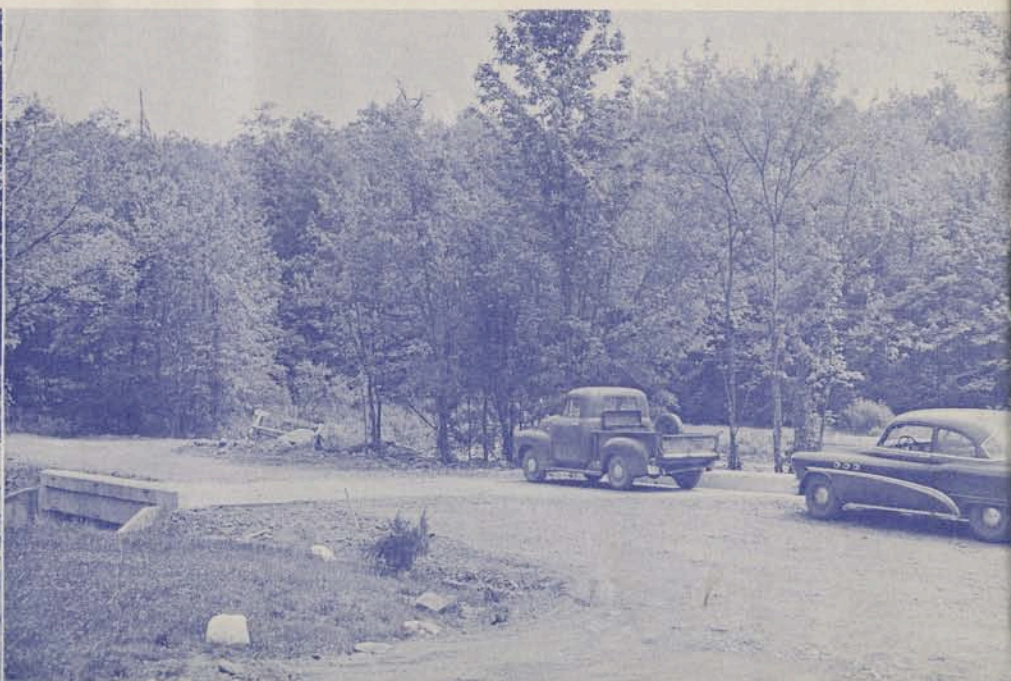
BULGERS RUN , east of Tannersville. Traffic Route 611. 11-foot masonry arch replaced by prestressed 22-foot span.
