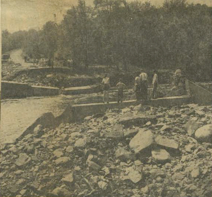
Sterling Creek changed its course north of the community. The wrecked amusement building at Toby Park on Route 115 near Blakeslee Corners is shown in the lower left picture. It was cut in half by the Tobyhanna River and swept over 100 yards from its original site. A concrete bridge for Route 940 across the Tobyhan-
