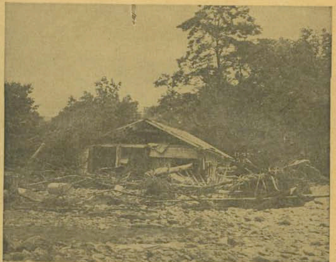
FAR FROM ORIGINAL LOCATION —The Valance Photo Studio, Canadensis, was lifted from its foundations in the heart of the town business district and deposited, amid a sea of debris, at a point 100 yards from its original location. As the height of the flood in that area water rose to a depth of over five feet.
