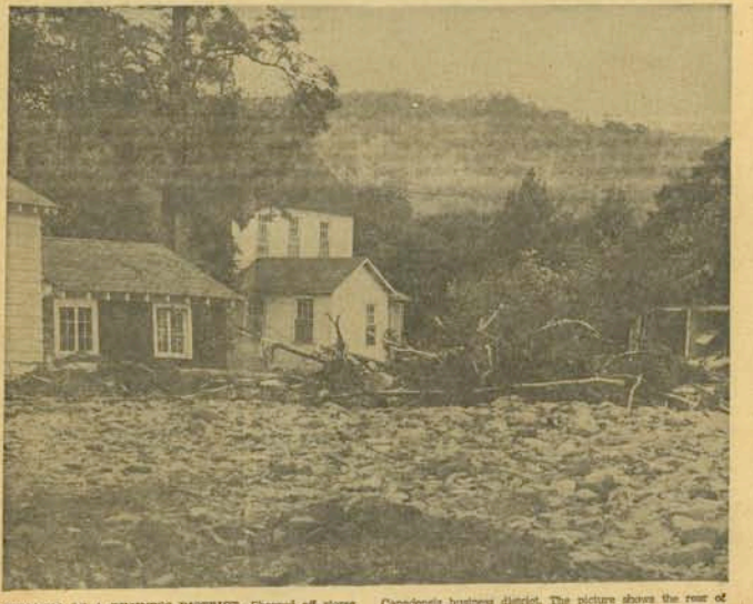
REMAINS OF A BUSINESS DISTRICT —Sheared off stores and battered business places give graphic evidence of the fury of flood waters which rumbled through the heart of the Canadensis business district. The picture shows the rear of the business section — a vast difference from its former orderliness.
