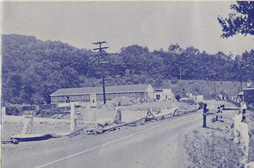
POCONO CREEK, Tannersville. Off Traffic Route 611. Masonry arch replaced by 60-foot I-beam bridge. Job completed.
