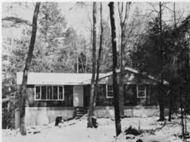
Mariano cottage under construction
