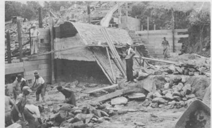
Building Dam for Lake Crawford
