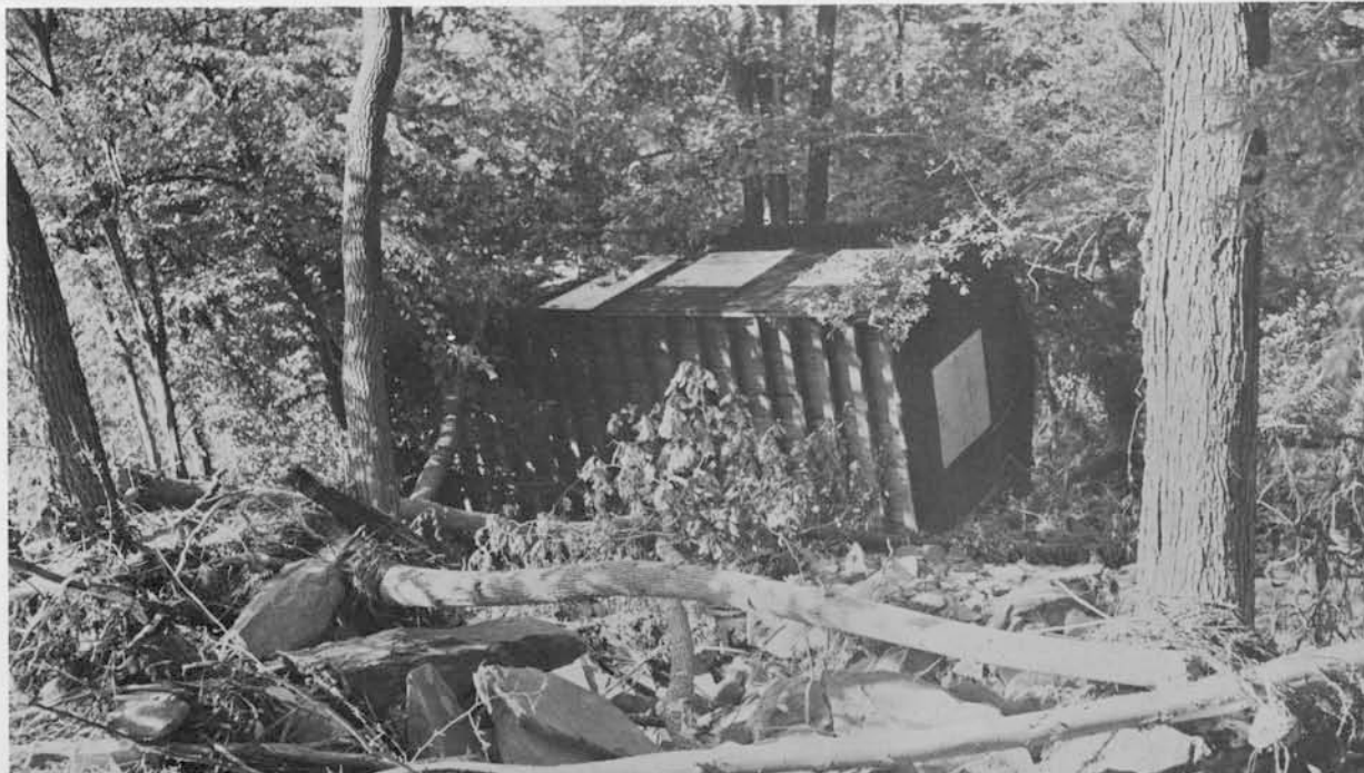
1955 Flood Damage at Girls' Camp
