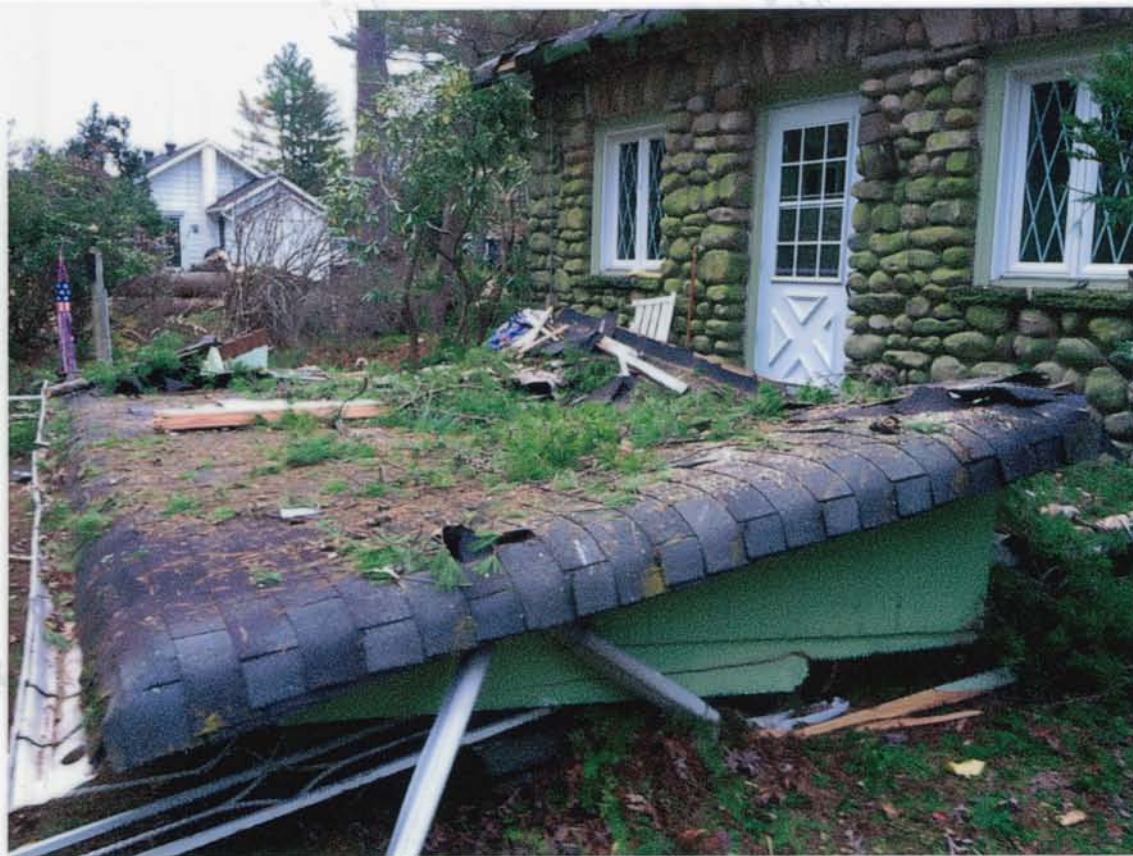
#45 Cottage owned by the Searings lost their front porch to the high winds of Sandy
