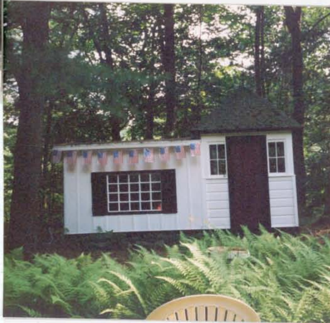
We're grateful to this cottage for preserving for posterity the old P.F Toll Booth which is the right half of their storage shed located to the left rear of their home
