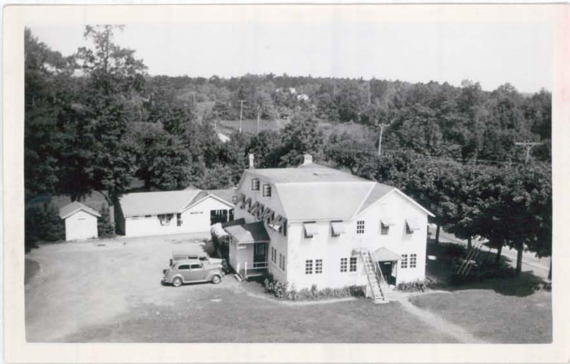
#3 Edition - Awnings, open attic windows cooled guests. First level bump-out bathrooms were popular convenience. Lattice work hid refuse area behind Gate Lodge kitchen.
