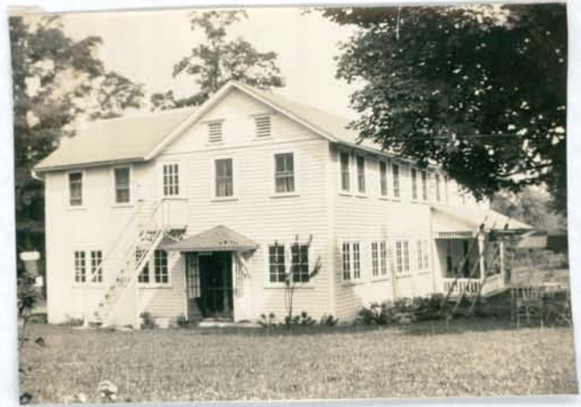
#2 Edition - A 2 story addition featured 8-10 guest bedrooms above and a Tea Room below. The exterior fire escape supplemented indoor office area staircase.
