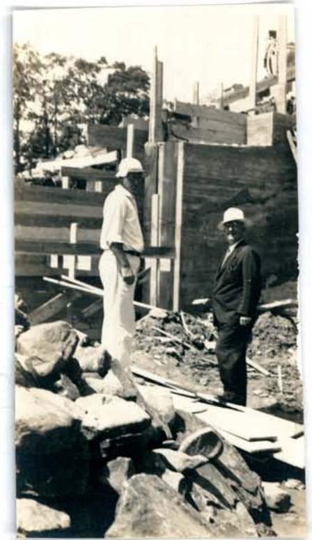
Left Harold Heydt (Caretaker) and Erwin Moyer (Manager) examine 1938 dam building
