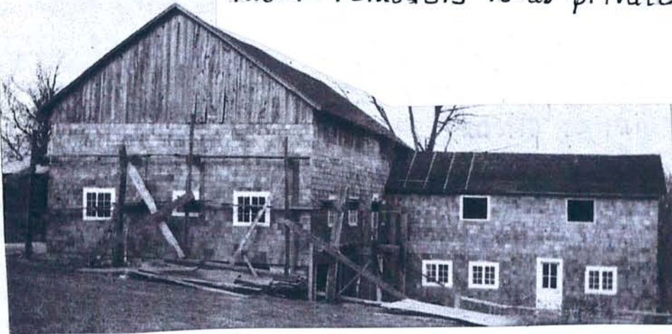
L-shaped Dimmick Dietrich barn under construction to become Nestledown Inn
