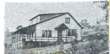
#25 home at base of dam
