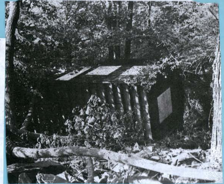
1955 Flood Damage at Girls' Camp
